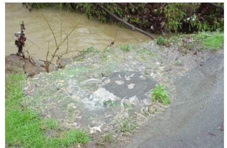
Wastewater overflowing down a busy street
